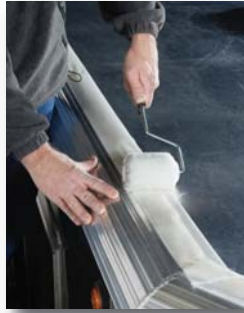
7 Roll down with a soft roller to conform over contours, seam edges, rivets, or screw heads.
