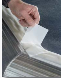
8 Peel off the protective release liner.
