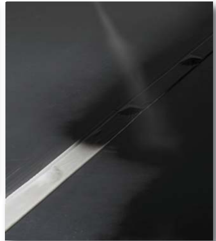
9 Burnish once more to optimize adherence and conformance to uneven surfaces.
